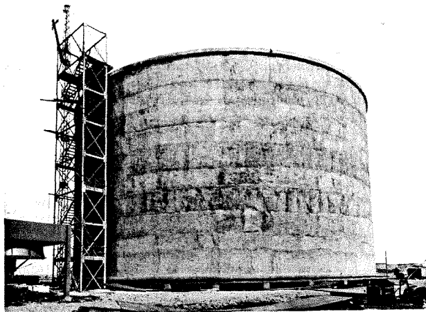
Figure 2. The ammonia storage tank under construction.
